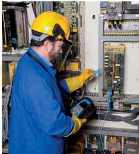
Operational testing on the electronic command-control part of a machine-tool.
