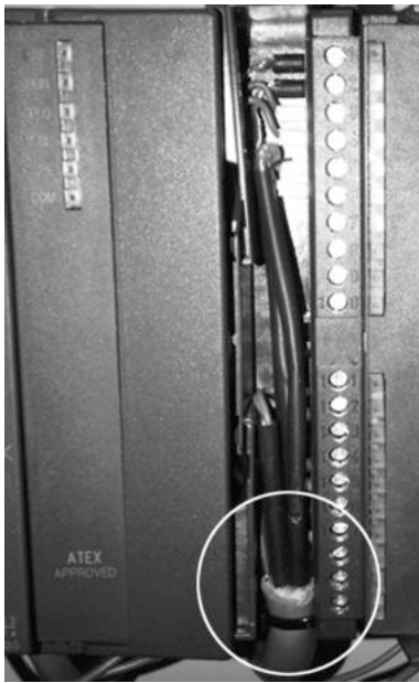
Figure 5-7 Correct sensor cable shielding
