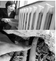
Heating Pipes/ Underfloor Heating Pipe Leaks
