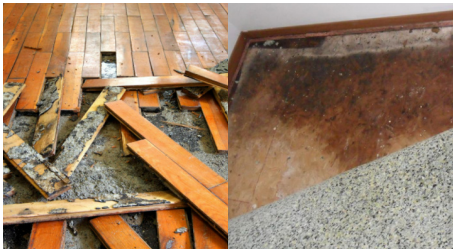
Leak Under The Floor
