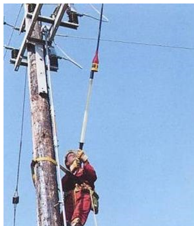
Overhead Line Testing
